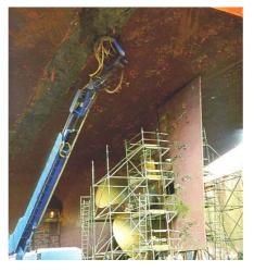
The blasting head can be swivelled so that both horizontal and overhead surfaces can be cleaned.
